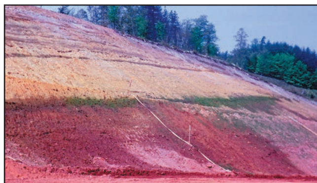
Figure 8. A cutting along the re-aligned A380 road exposing the boundary between the yellow-brown Upper Greensand and the underlying red Teignmouth Breccia.
